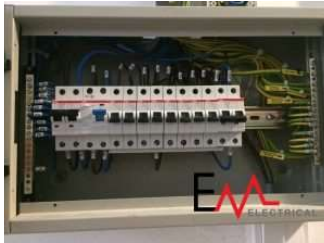
Figure 13. Correct circuit breaker installation
