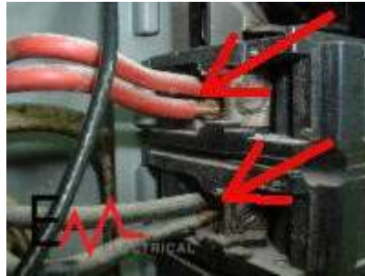
Figure 24. Loose Connections
